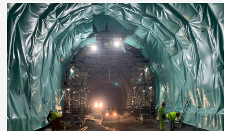
2mm PVC liner installed in the arch structure
