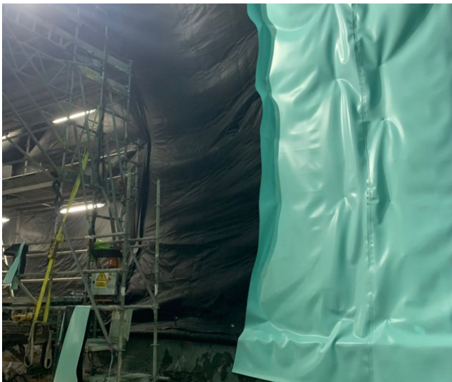
Installing the PVC membrane from the inside, connected to the EnkaDrain.
