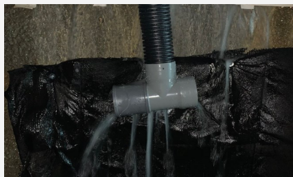
Infiltrating water collected by EnkaDrain
